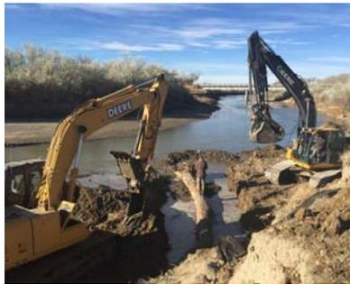
prone bench and the upper terrace were reconstructed, both areas were seeded and approximately 2,902 square yards of turf reinforcement mat and erosion control mat was installed.
