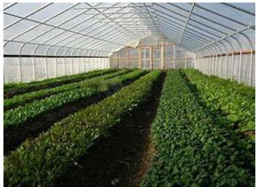
The high tunnel structure must be planned, designed, and constructed from a manufactured kit in accordance with manufacturers' recommendations. The high tunnel frame must be constructed of metal, wood, or durable plastic; and be at least 6 feed in height at the peak of the structure. The high tunnel covering material shall have a 4-year-minimum lifespan. For polyethylene covers, a minimum 6-mil greenhouse grade, UV-resistant material should be used.
